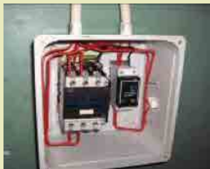
Lights timer set to switch on at 5h30 and switch off at 19h00
